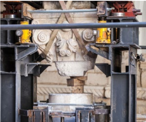
REPAIR OF CHAPTERS IN THE RECTOR'S PALACE Source: Institute for the Restoration of Dubrovnik
